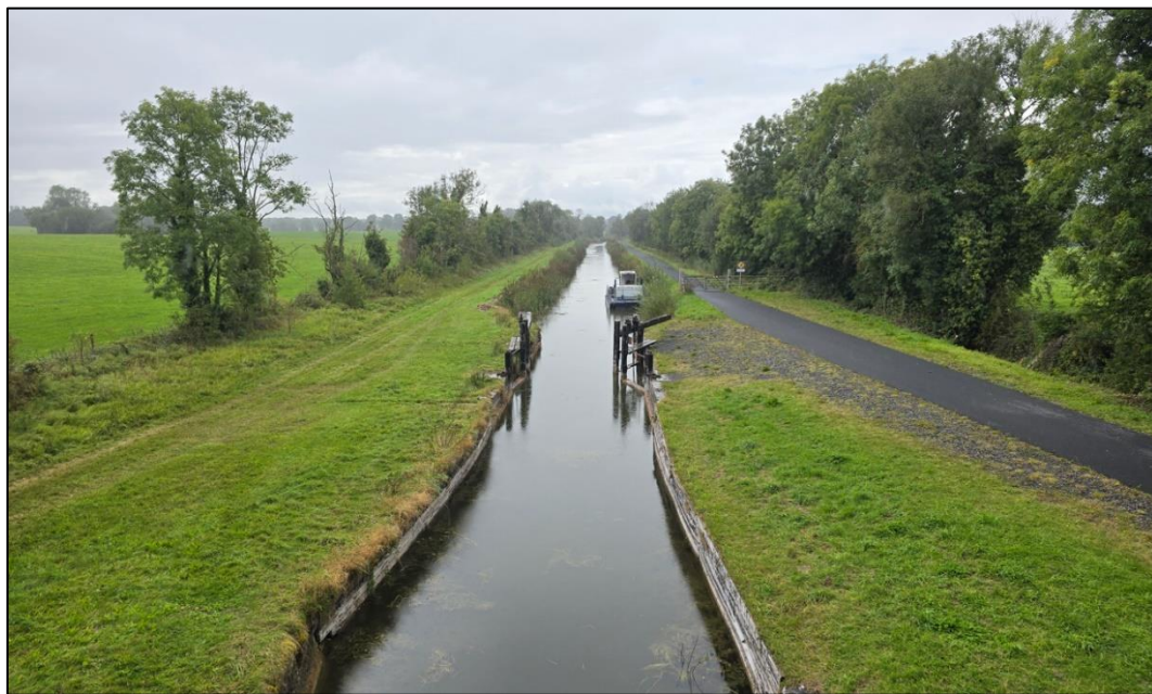
Figure 3-4: View of Grand Canal from Rathmore Bridge to East of Crossing Location
