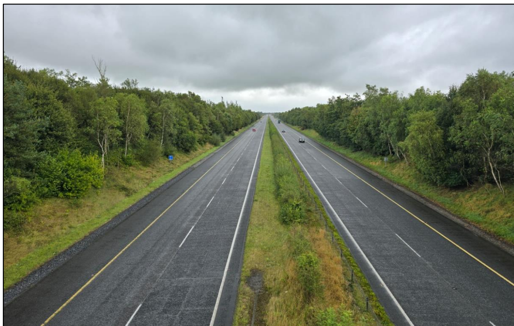
Figure 3-2: View of Carriageway from Bridge Structure at M4 Motorway Crossing
